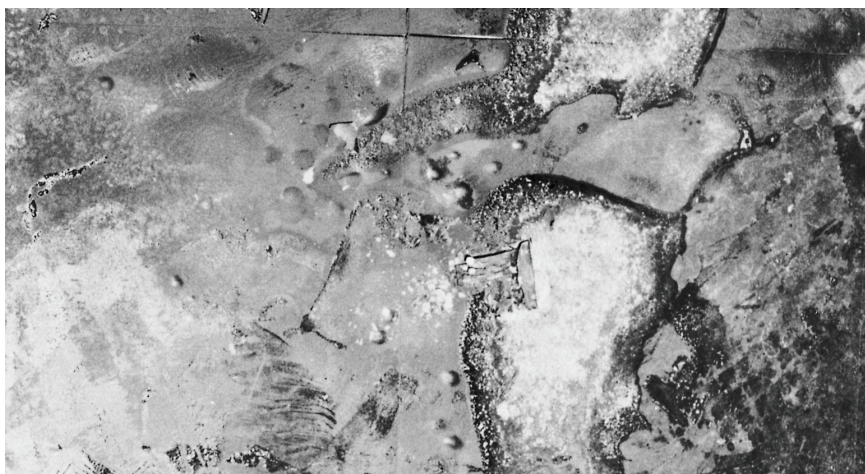
Fig. 31-2 Char pattern typical of the use of accelerants. The area where the accelerant is in contact burns hotter and therefore leaves a char pattern that is different from surrounding areas. Door propped open, holes chopped in floors, "trailer" used to direct the fire from one area to another, etc., are all reasons to suspect that a fire is due to arson.
